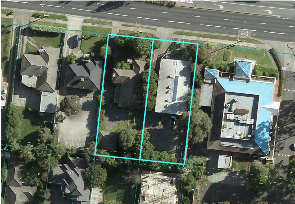
Figure 2 – Site Aerial Photo (16 March 2020)
