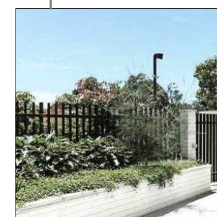
DARK GREY PAINTED PALISADE FENCE
