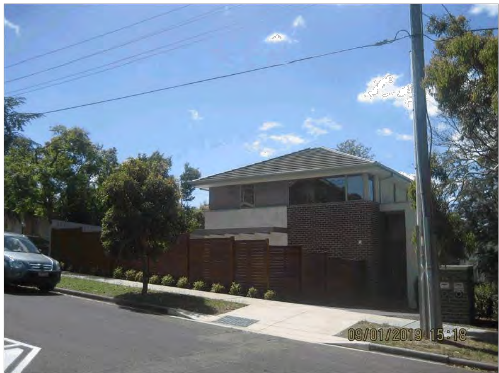
The front of the 3-unit development at 19 Glendale Avenue, immediately to the west of the subject land.
