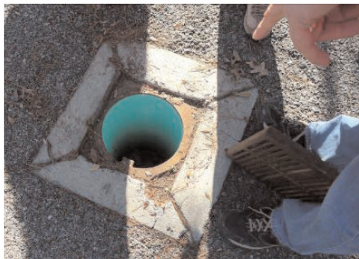
Figure 16- Observation well enables inspection of water infiltration
