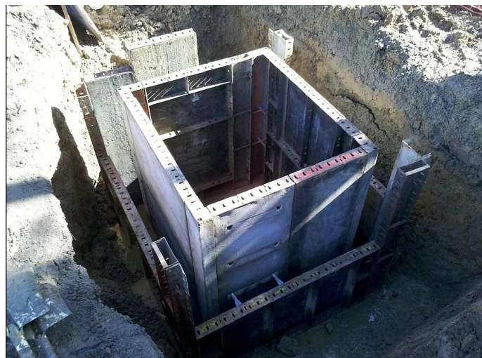
Figure 2 - Junction pit construction
