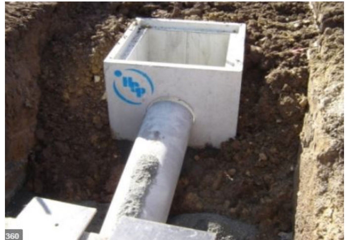
Figure 3 - Outfall drain construction
