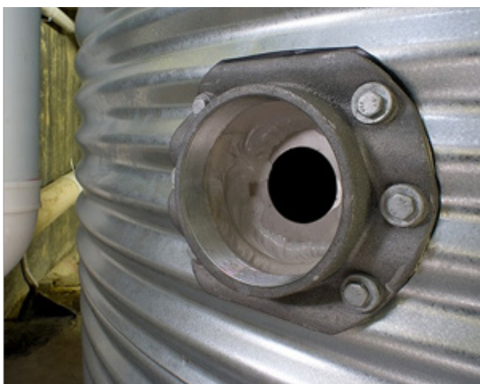
Figure 5 - Rainwater tank orifice installations
