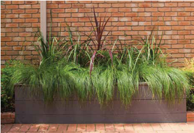
Figure 10 - Planter box raingarden
