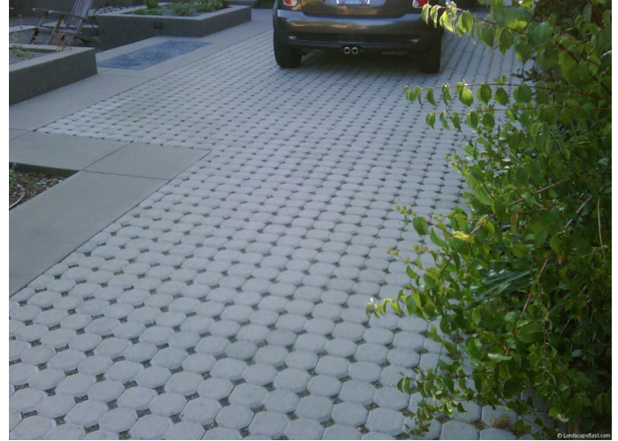
Figure 12 - Modular block systems
