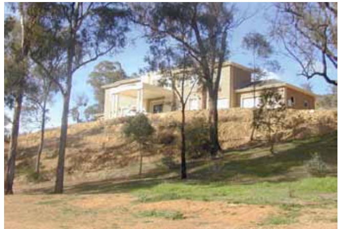
Excessive batters are hard to manage and are susceptible to erosion
