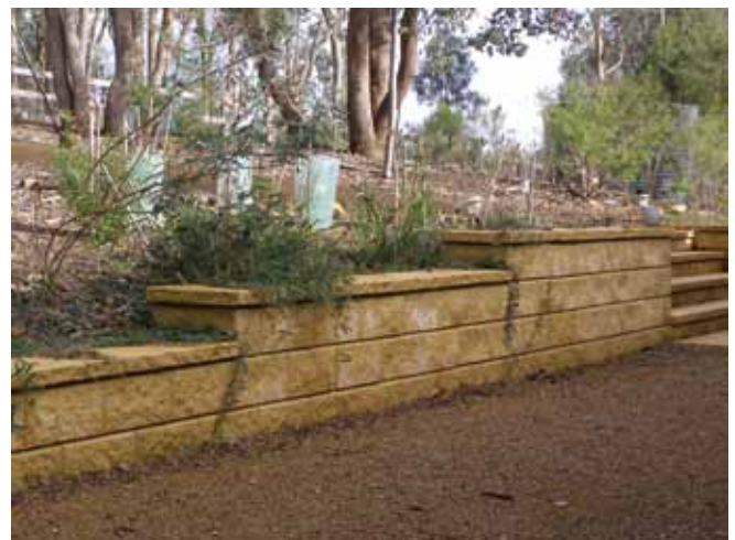
Retaining wall secures the cut and reduces erosion
