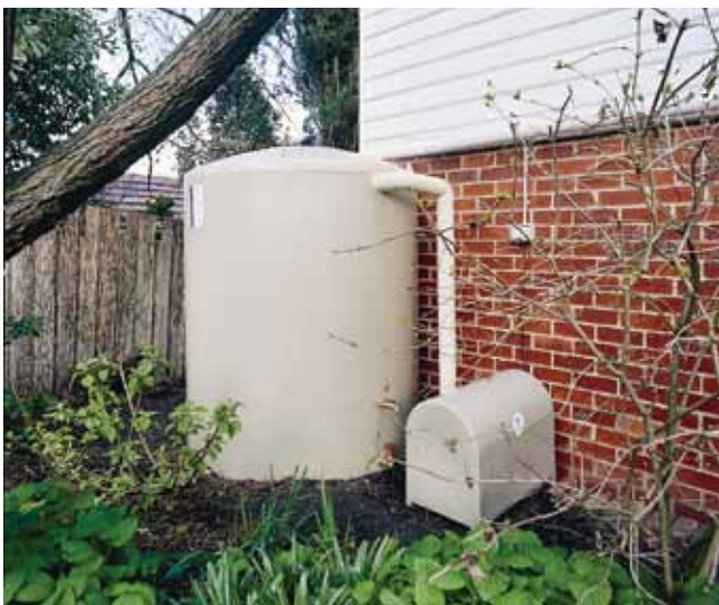
Water tank with pump cover to protect the pump and reduce noise
