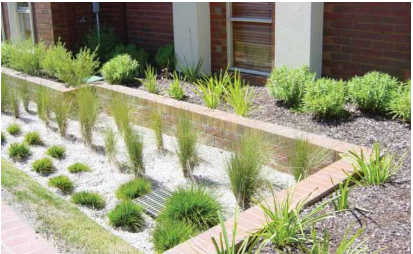
Example of a raingarden
