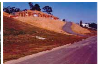
Poor example of development, using excessive fill
