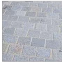
PORTE COCHERE ENTRY PAVEMENT BLUESTONE PORPHYRY SETTS
