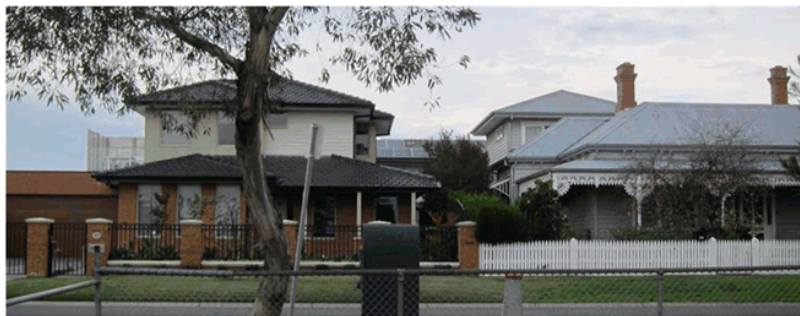
Figure 3 Existing dwellings on the Site 2
