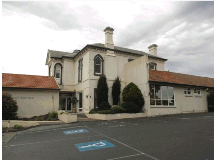
Figure 1 West elevation of Tullamore, with later single-storey additions
