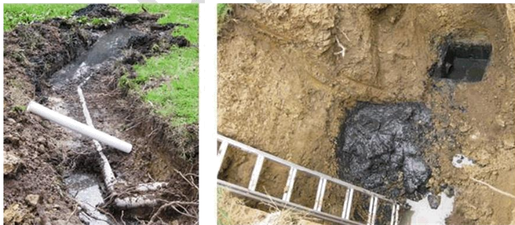
Figure 11: Flooded irrigation field and a deeply buried distribution pit (legacy system)
