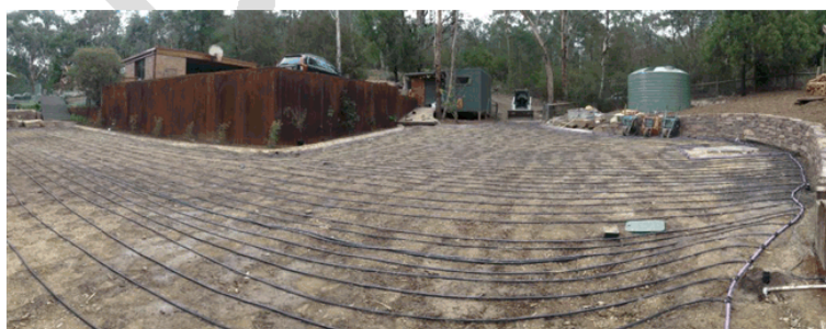
Figure 4: Lay-down of sub-surface irrigation
