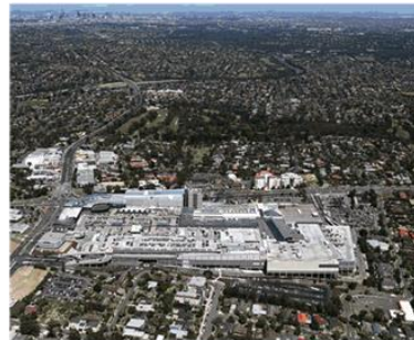
Figure 23: Aerial view of Westfield Doncaster showing sloping nature of Doncaster Hill and views towards Melbourne CBD west of the site.
