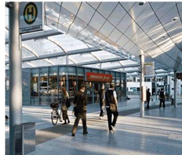
Figure 40: Upgraded and relocated bus interchange to enable direct access to Williamsons Road, entry forecourt and complex and improved bus and pedestrian environment.
