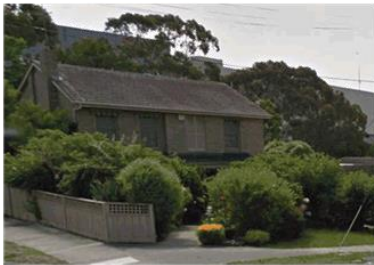
Figure 92: Existing double storey dwelling on Roseville Avenue
