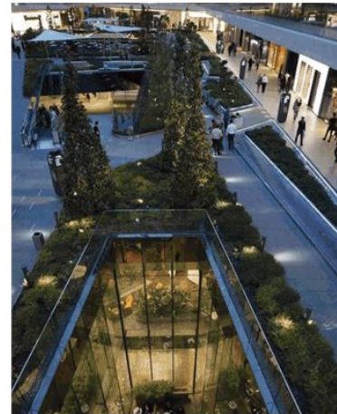
Figure 48: Potential to establish an upper level dining terrace to activate upper levels and establish activity on Williamsons Road.
