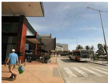
Figure 26: There is little engagement between the primary pedestrian entrance and the bus interchange
