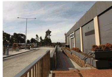
Figure 16: A significant built form setback from Williamsons Road provides limited engagement with the street and results in an undefined northern gateway to Doncaster Hill.
