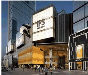
Figure 44: An example of an articulated, high-quality forecourt and entry visually marking the key entry into the retail centre.
