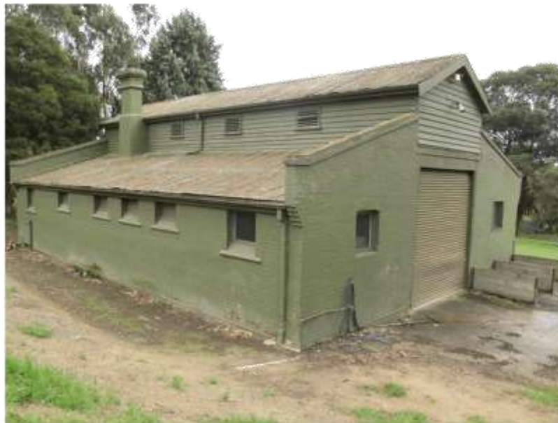
Figure 4 South and east elevations of the stables building.
