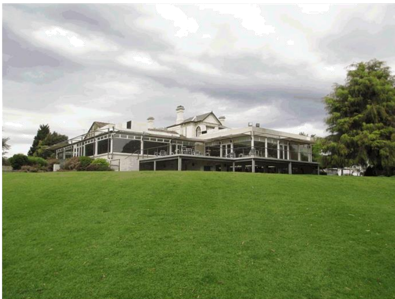
Figure 16 View to the clubrooms from the north-east. The first floor of the original homestead is visible above the later single-storey additions.
