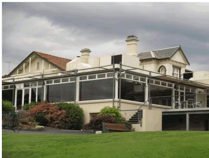
Figure 2 View towards Tullamore from the east showing the clubhouse additions
