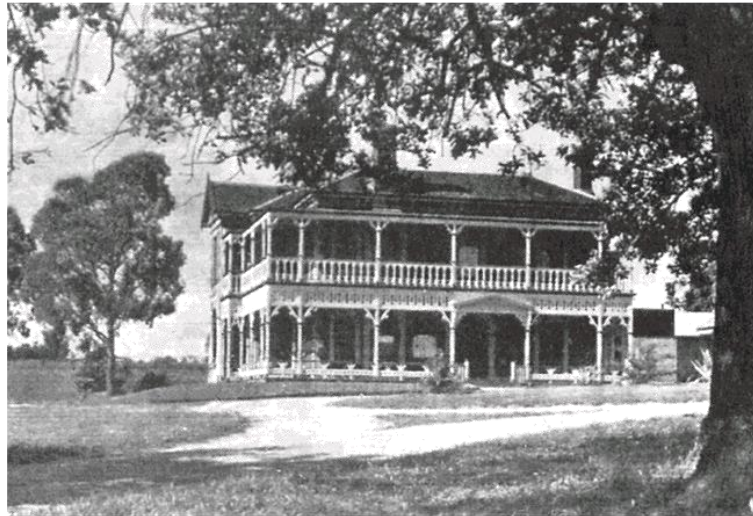
Figure 2 Early view of Tullamore homestead, showing the original two-storey timber verandah to its north and west sides. Source: The History of the Eastern Golf Club, p. 9.
