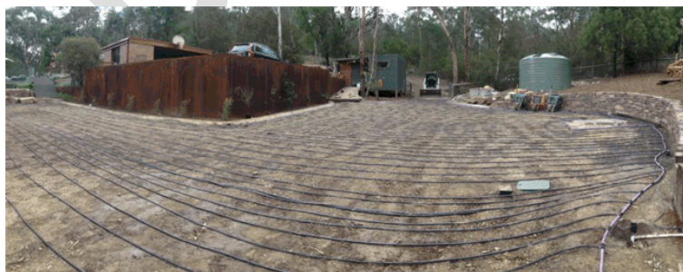
Figure 4: Lay-down of sub-surface irrigation
