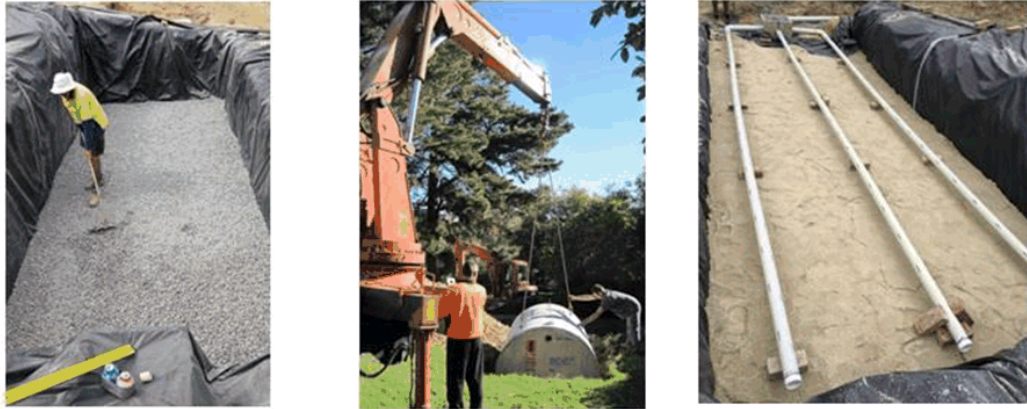
Figure 3: Septic system components in various stage of construction/installation
