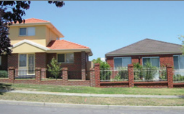
Step upper levels back from boundaries to integrate development with single storey streetscapes.
