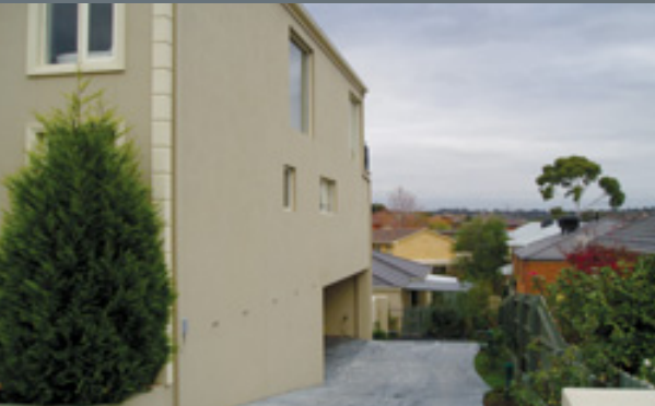
High floor levels and the lack of stepping with the slope will emphasise building height and bulk.
