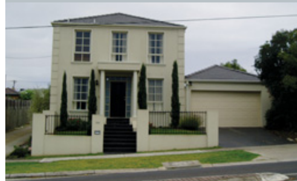
A symmetrical presentation and vertical elements can emphasise the visual prominence of a dwelling.
