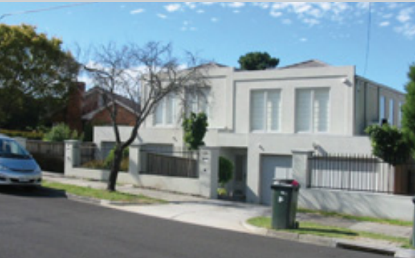
Uncomplimentary roof forms add to building bulk.
