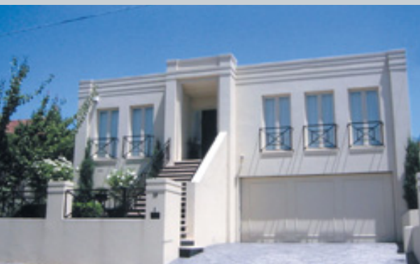
High parapets and lack of visible roof line can exaggerate building height and bulk.
