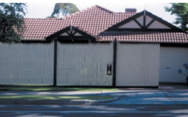
High front fencing obscures development and landscaping and may create security problems.
