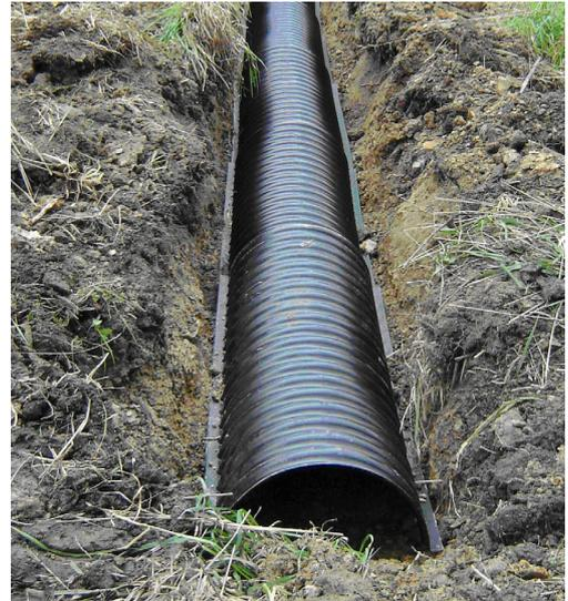
There is a concrete distribution pit (or 'box') at the start of the first trench (and sometimes at the start of each trench). Effluent is distributed evenly throughout a trench, which must fill to approximately 150mm below ground level before overflowing to the next trench, via a 'weir', or 'overflow'. Trenches are typically a minimum of 10m, and a maximum of 30 meters long.
