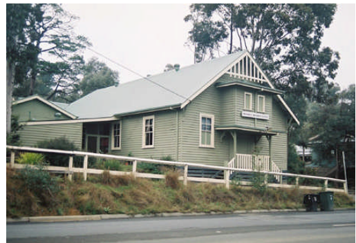
The Mechanics Institute in Yarra Street
