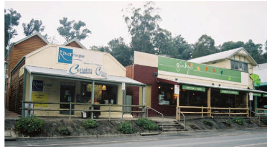
Retail buildings in Yarra Street
