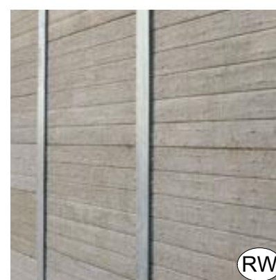
CONCRETE RETAINING WALL - WOOD GRAIN FINISH
