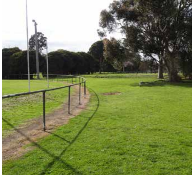
The sportsground at Koonung Park – new cyclone mesh fence is one of the new features proposed as part of the management plan.
