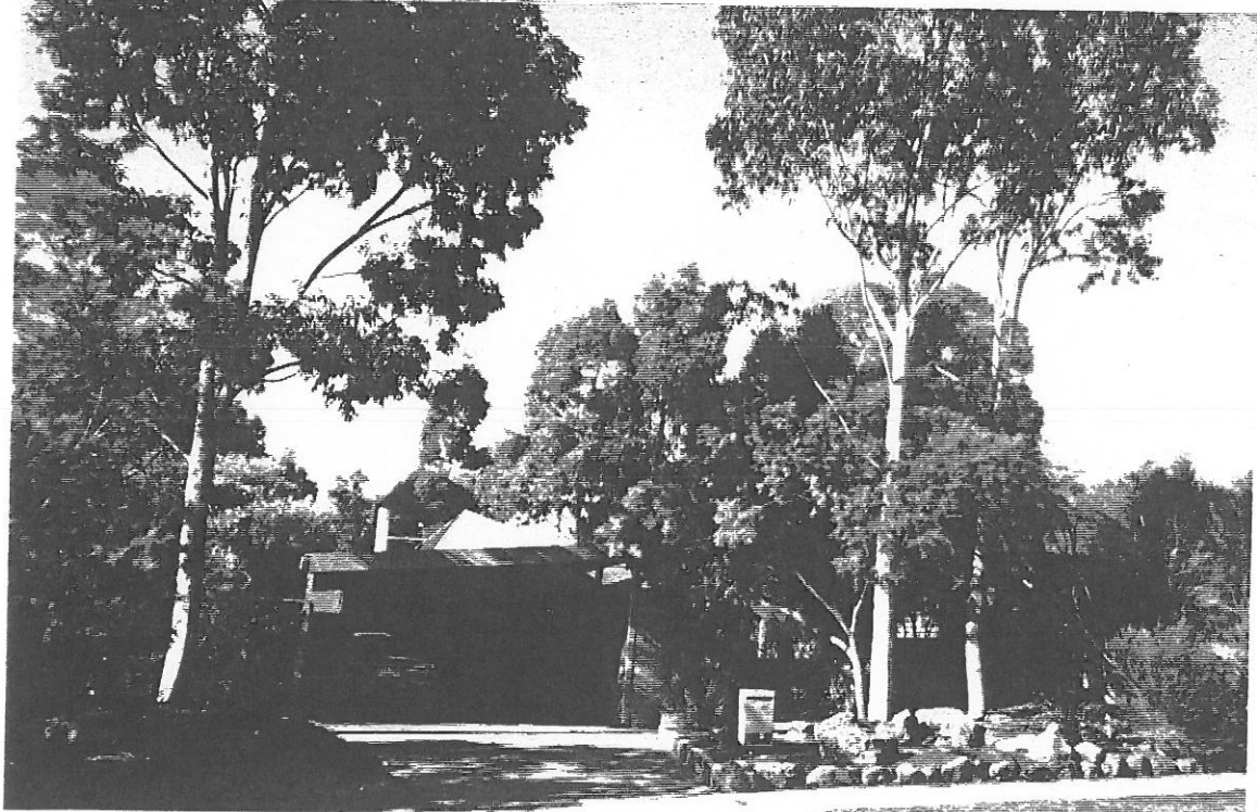
32 ROSCO DRIVE (SOLAR HOUSE)
