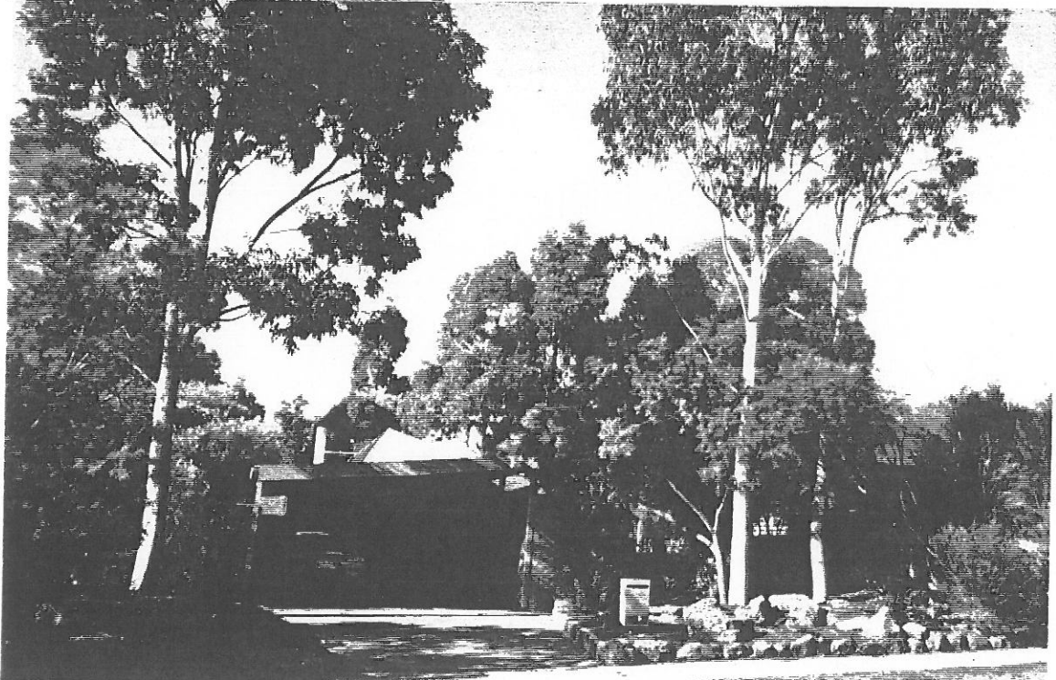
32 ROSCO DRIVE (SOLAR HOUSE)
