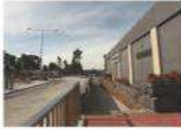
Figure 22: A new public space with a paved walkway, benches, and greenery.
