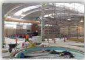
Works continue at Aquarena
