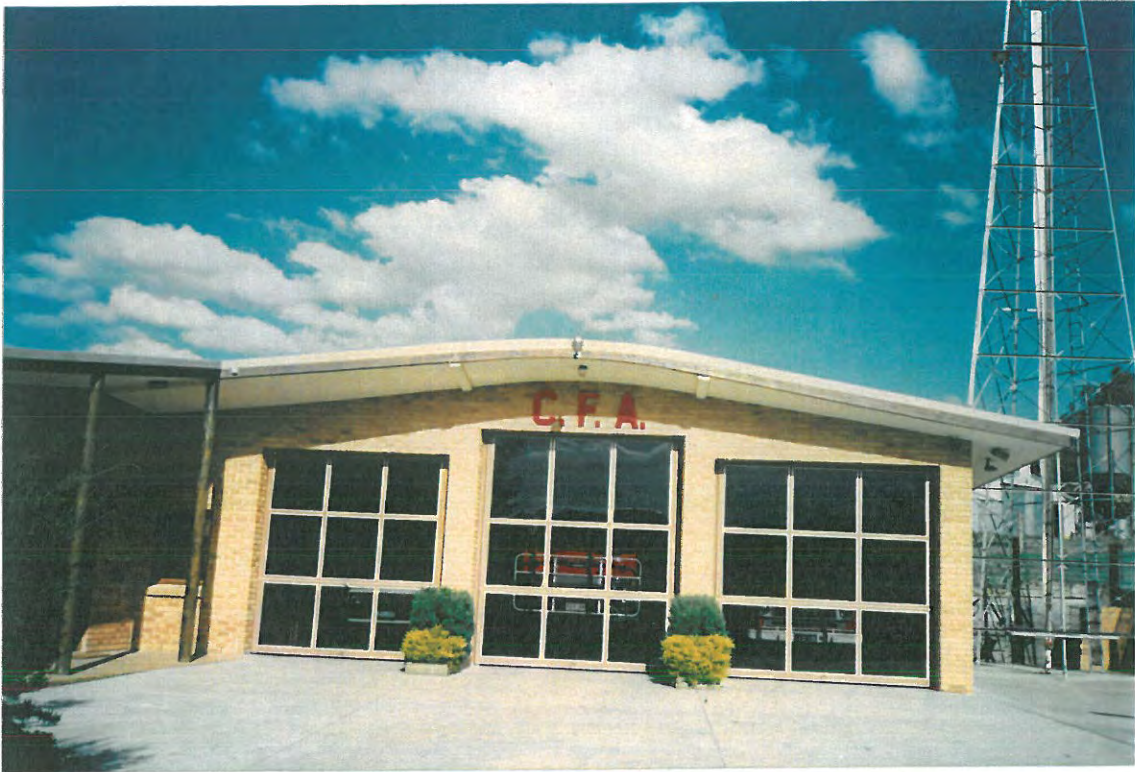
South Warrandyte Fire Station, Brumbys Road, Warrandyte
