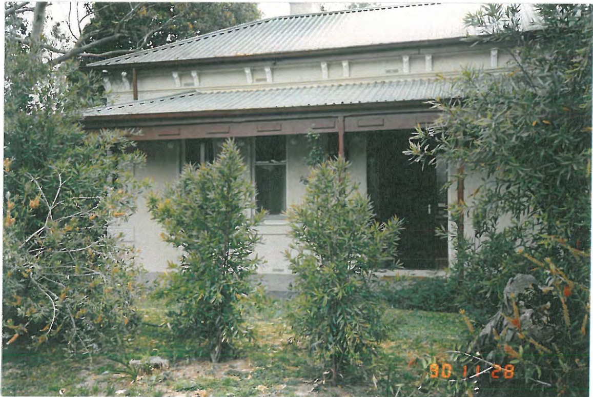
House, 88-90 George Street, Doncaster
