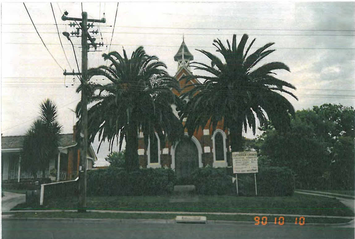
Trinity Lutheran Church, 53 Victoria Street, Doncaster
