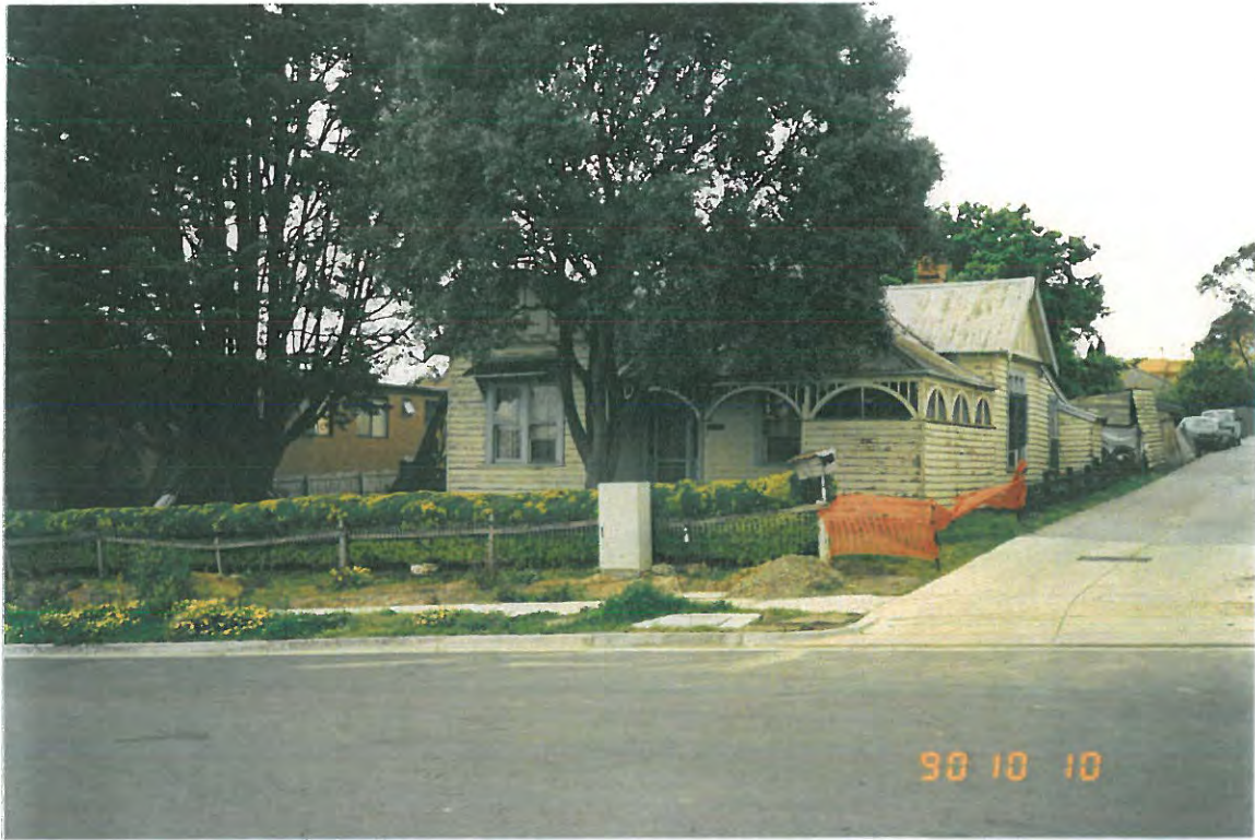
House, 4 Beaconsfield Street, Doncaster
