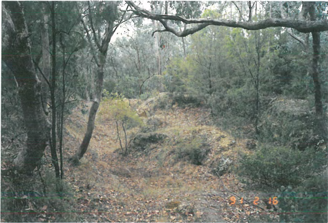
Black Flat Mining Area: the collapsed 'dyke'
