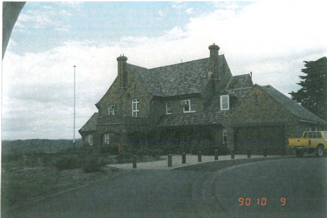
Westerfolds Manor, Westerfolds Park, Templestowe
