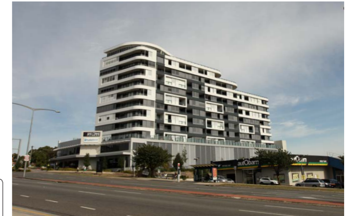
Figure 14: Recently completed apartment building with 12 storeys built form height along Doncaster Road
