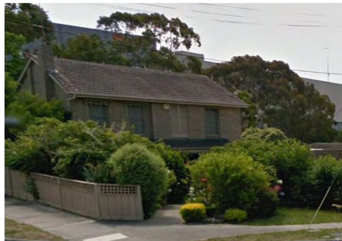
Figure 70: Existing double storey dwelling on Roseville Avenue
