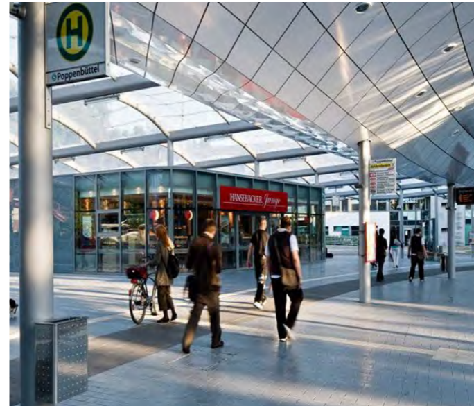
Figure 38: Upgraded and relocated bus interchange to enable direct access to Williamsons Road, entry forecourt and complex and improved bus and pedestrian environment.
