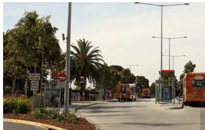
Figure 18: Buses entering and exiting the bus interchange may conflict with vehicular transport, limiting efficiency and reliability of services.
