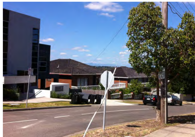
Figure 65: Residential dwellings along Westfield Drive are single or double storey in height establishing a low-lying residential interface to the north
