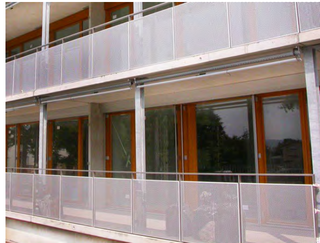
MP-2 METAL PANEL COLOUR 2 PERFORATED ANODISED ALUMINIUM
