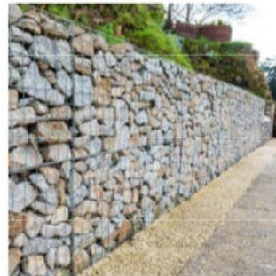
c) Gabion wall
