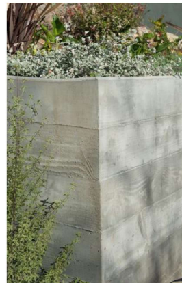
Potential retaining wall options: a) and b) in situ concrete with timber form work
