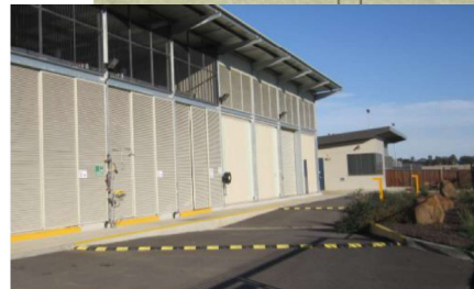
Example of spill capture bund within roadway
