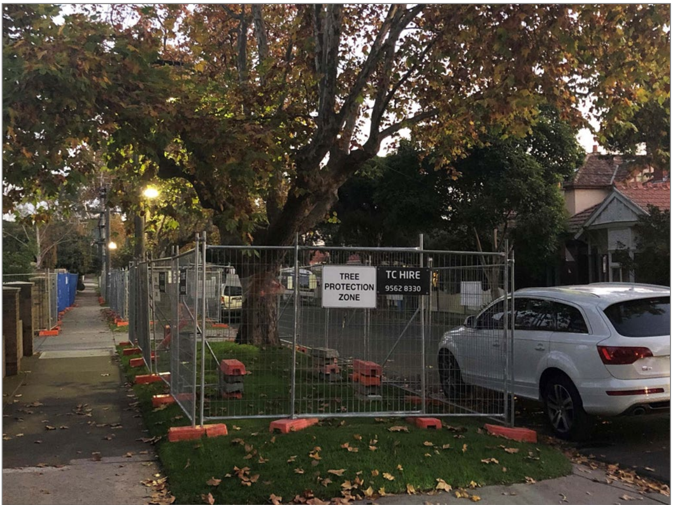
10. Example of tree protection fencing for establishment on nature strip (Photograph courtesy Susan Murphy, Urban Tree Planner City of Boroondara, May 2021) Public Tree Removal
