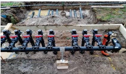
Deep Creek Irrigation (in progress)
