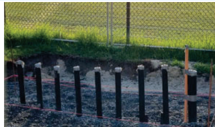
Koonung Reserve Irrigation (in progress)
