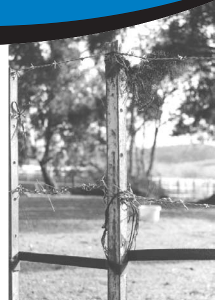
A survey of horse injuries showed that one in six injuries were caused by a fence or a gate. Improving your fencing is a worthwhile investment.
