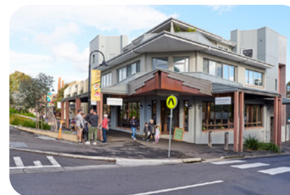
Figure 28. Shoptop housing, Eltham
