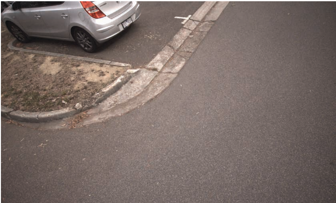
Figure 21 Snapshot of a very poor Kerb and channel in Anderson Park off-street carpark.
