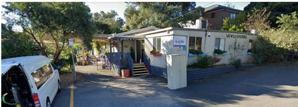
Figure 9 – KHG Office Building (shown in Figure 3 as Building 7)
