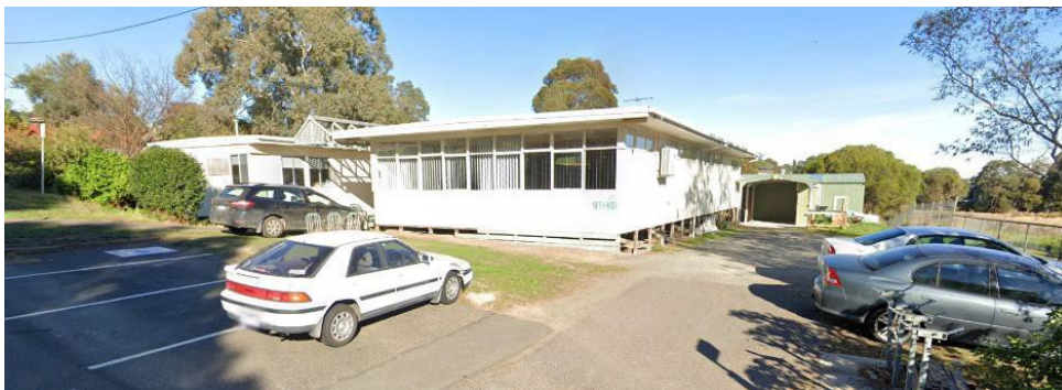
Figure 8 – Manningham Men's Shed (shown in Figure 3 as Building 18)
