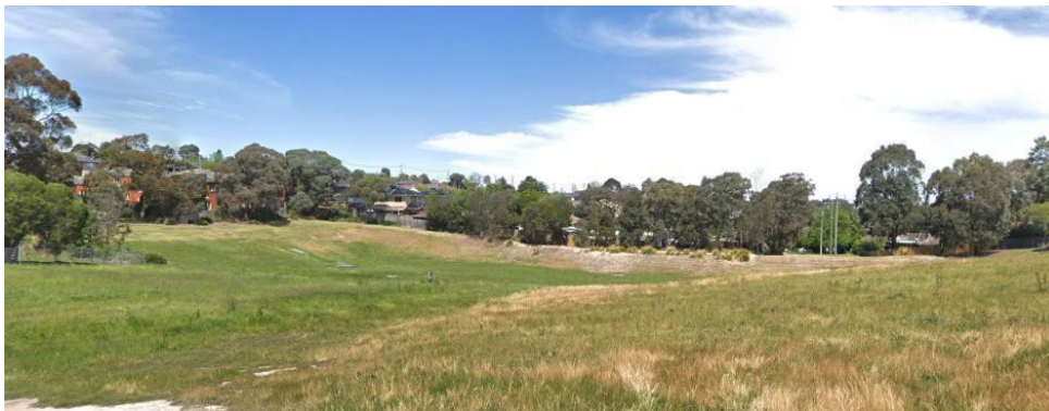
Figure 21 – Drainage detention basin on north side of the bank (additional drainage basin on south side of bank with access from Coolabah Street)
