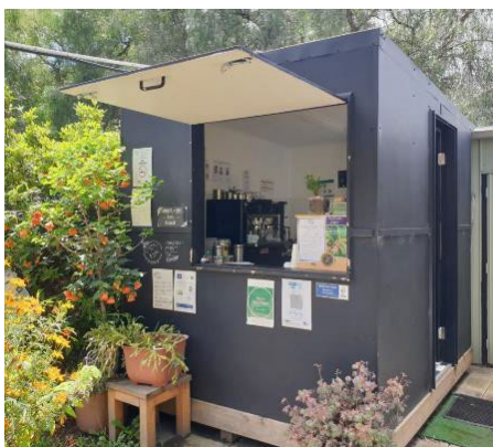
Figure 25 – Example of relocatable hut profile. This is KHG's Peppertree Place café at the Coburg Campus
