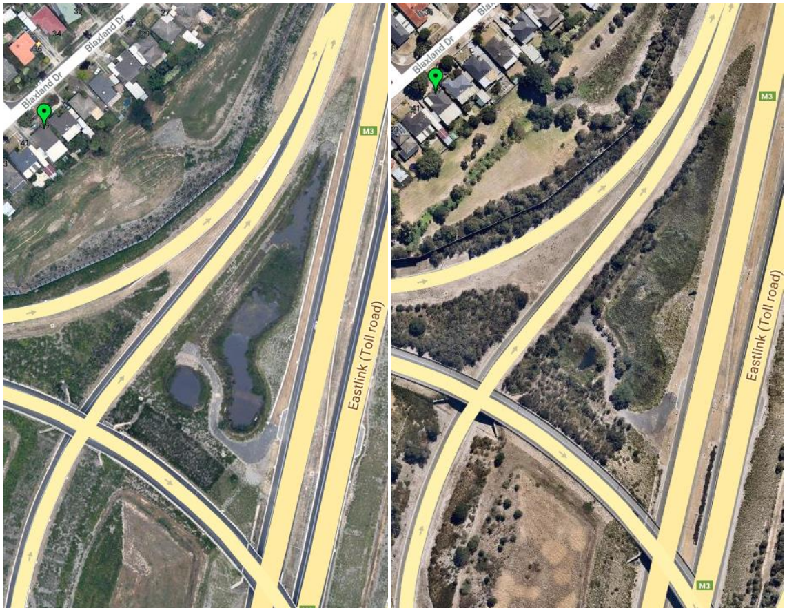
Appendix E 6 East Link Sediment Ponds (Monash Freeway) November 2009 (left) and February 2019 (right)
