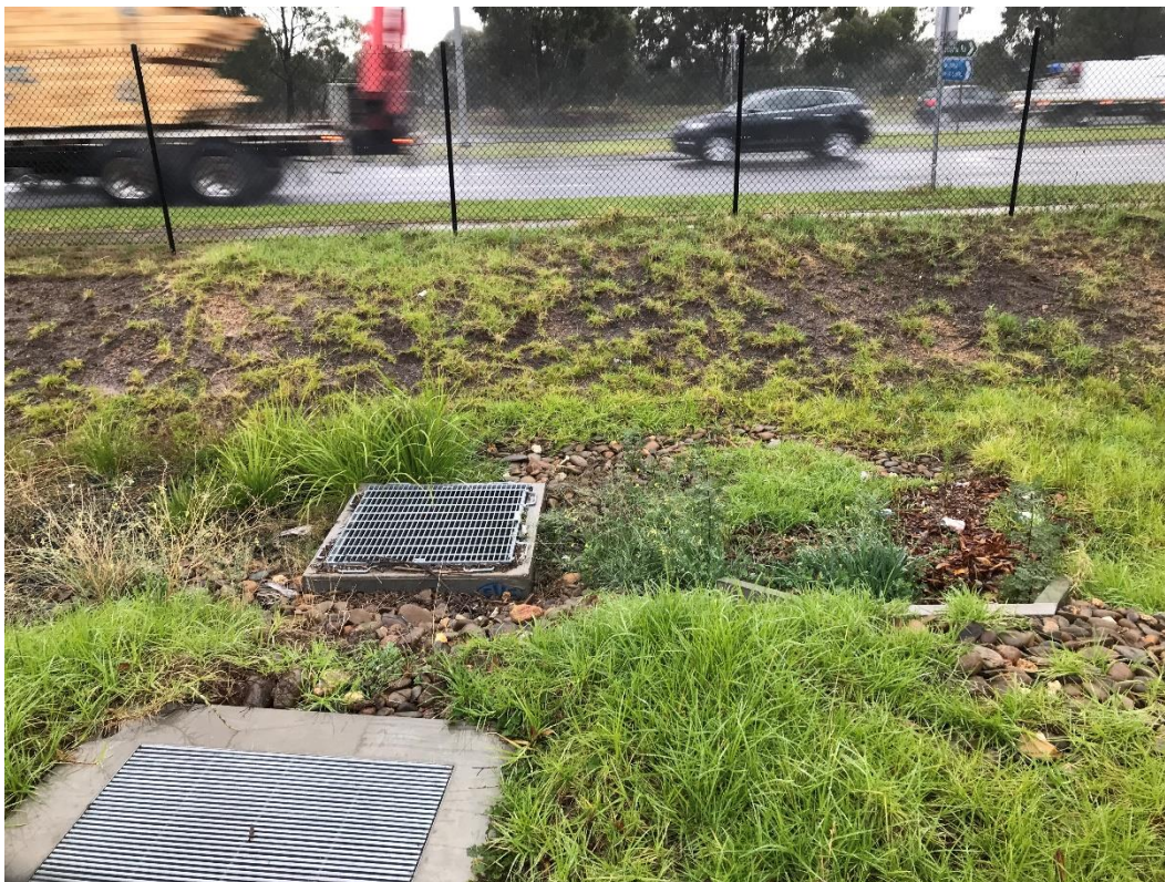
Appendix C 5 Existing basin within Watsonia Railway Station carpark
