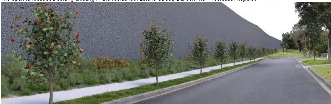
The proposed expansion of the Freeway corridor and new 10m high noise attenuation walls. Ref -Technical Report H
