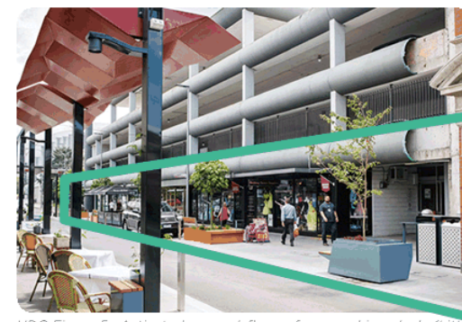
UDG Figure 5. Activated ground floor of car parking deck (Little Malop Street, Geelong)
