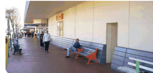
UDG Figure 21. Coles Wall - before activation (Wodonga)
