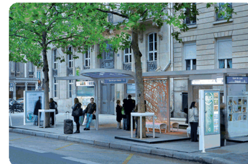
Figure 31. Enhanced bus stop design with public art and lighting, Gare de Lyon Diderot, Paris
