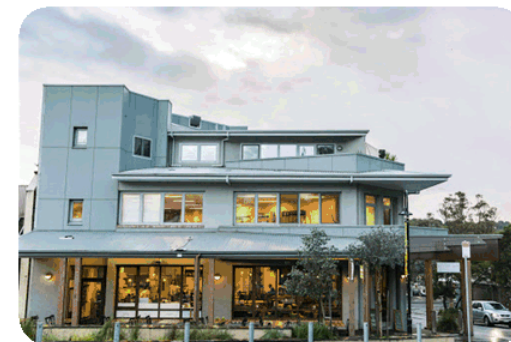
Figure 6. Shop top housing with commercial below, Eltham
