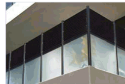
F11 1M HIGH OBSCURE GLASS BALUSTRADE WITH 0.7M HIGH BLACK LOUVRE SCREENING ABOVE. LOUVRE SCREENING TO HAVE NO MORE THAN 25% TRANSPARENCY.
