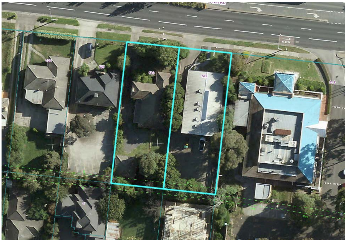
Figure 2 – Site Aerial Photo (16 March 2020)
