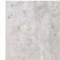
7 Light Concrete - Driveway
